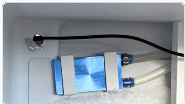
Correct position on the evaporator
